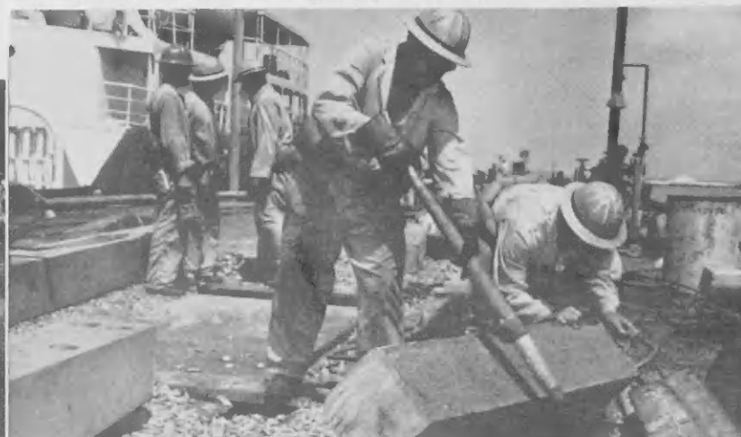
BEFORE DOWELS cover the openings, the area must be drilled to size, far left, and the bolt covered, left. The twelve-by-twelve-inch timbers are picked up and positioned by a crane after the bolt and dowel holes have been drilled. Holes are visible in the timber above.
